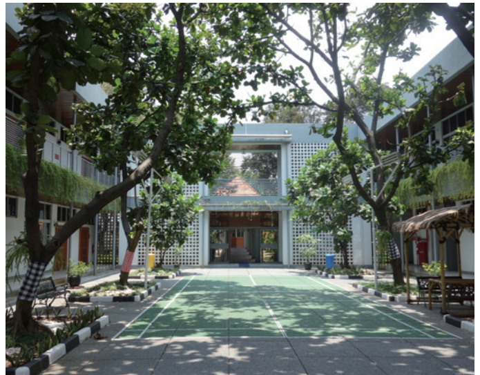
The Water Supply and Environmental Sanitation Training Center (WSESTC) today
