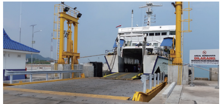
Merak Ferry Terminal
