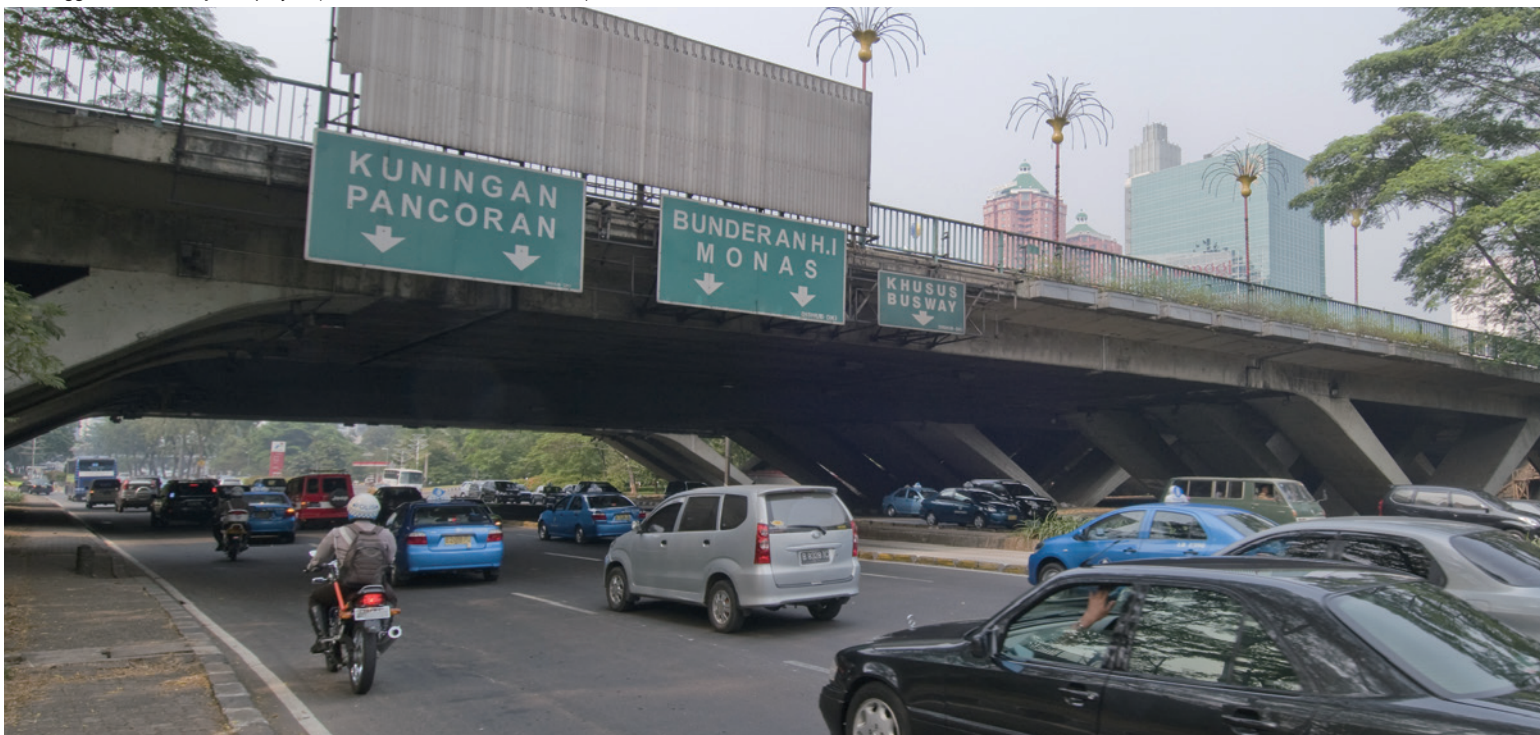
Semanggi intersection flyover project (Photo: Kenshiro Imamura/ JICA)
