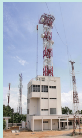
VTS Center in Batu Ampar (Photo: Japan Radio Company)
