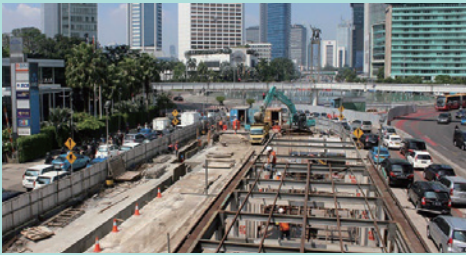
1: Construction near Bundaran HI Station
