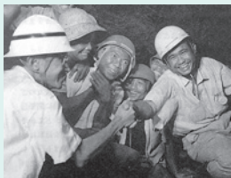
Engineers pleased with completion of excavation of the dam diversion tunnel (Brantas River Basin Development) (Photo: Nippon Koei Co., Ltd.)
