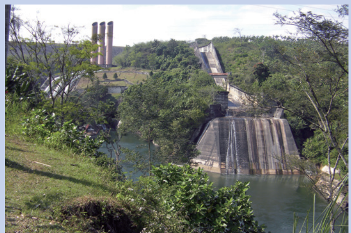
Karangkates Dam (looking up from downstream) (Photo: Nippon Koei Co., Ltd.)
