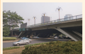
Semanggi intersection flyover project (Photo: Kenshiro Imamura/JICA)
