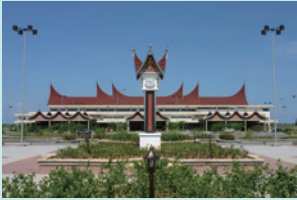
Passenger terminal building (Photo: Lukman F. Laisa)
