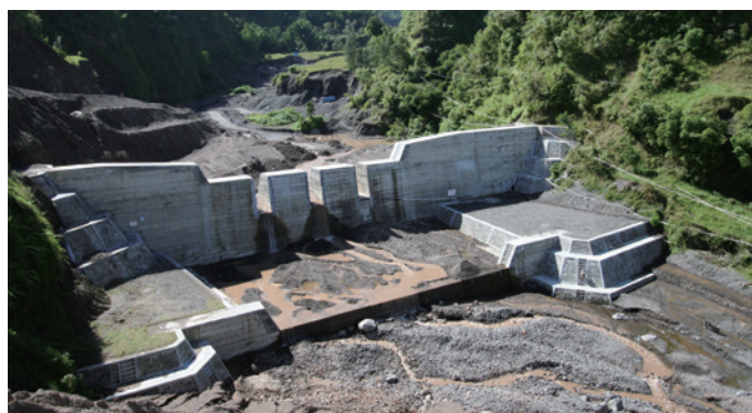
Sabo dam constructed by Japanese ODA loan (Photo: Yachiyo Engineering Co., Ltd.)
