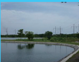
Wastewater treatment facility in Denpasar (Photo: JICA)
