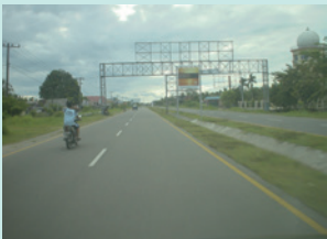
Airport access road
