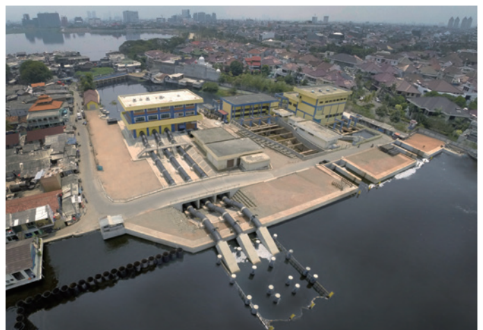
Pluit East Pump Station (Photo: JICA)
